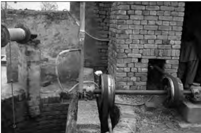
Photograph III: Tube well with uncovered shaft & belt
